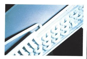
35. Insufficient load on the evaporator prevents all the liquid from vaporizing causing liquid flood-back unless an accumulator or other protective device is installed. There are many reasons for low load such as low or no air flow due to dirty filters, air restriction, air bypass, dirty fan wheels, loose or broken fan belts, and malfunctioning motors. Under these conditions the coil tends to frost and even a properly sized expansion device will tend to hunt.
